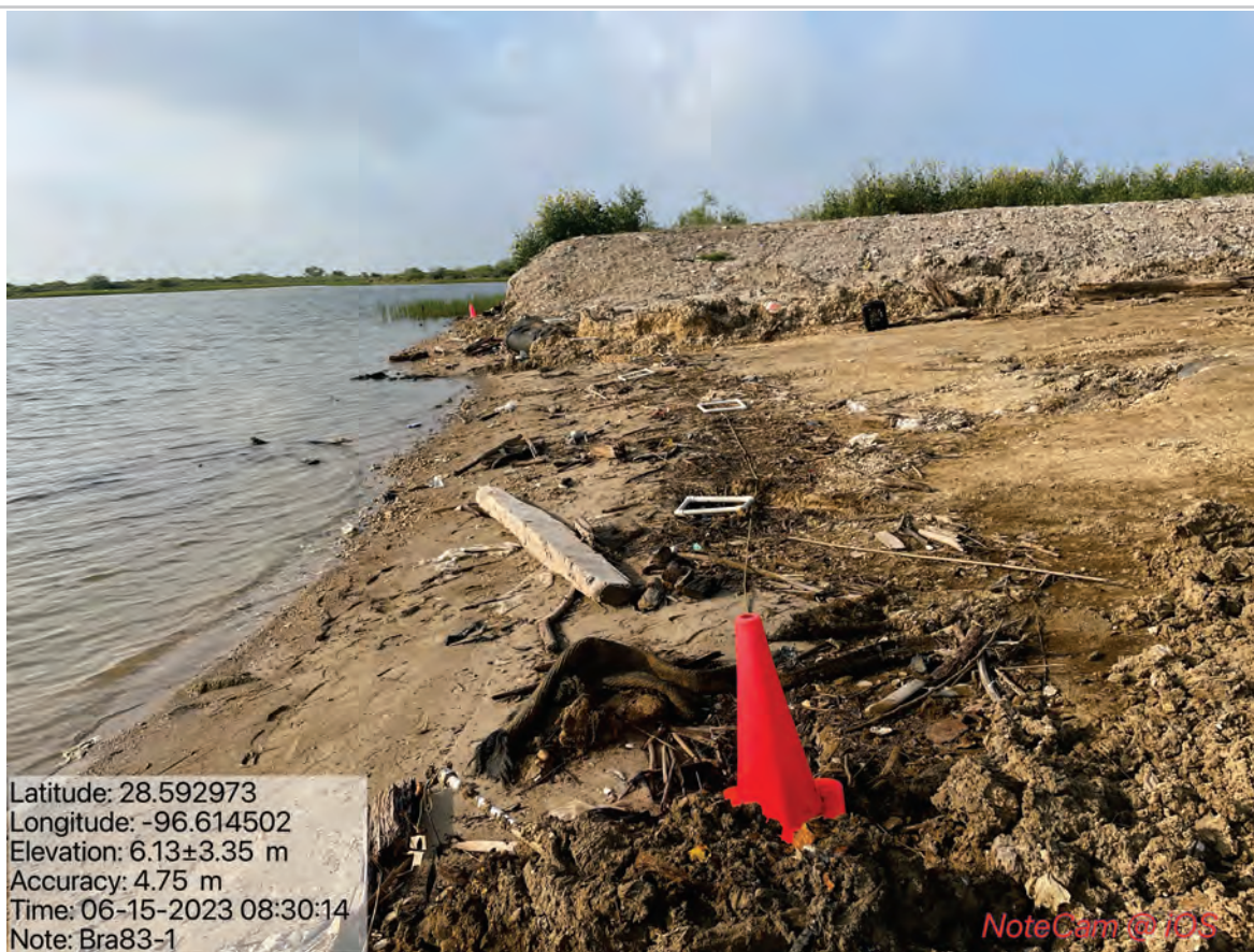
Shoreline AFTER interim bay cleanup activities.
