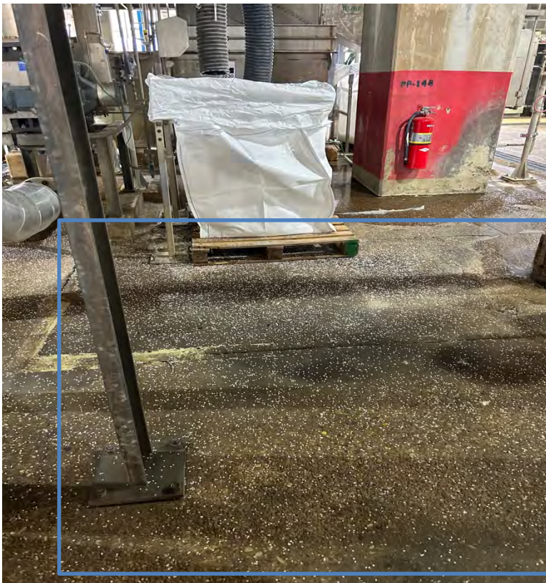
Extruder building B: Before
