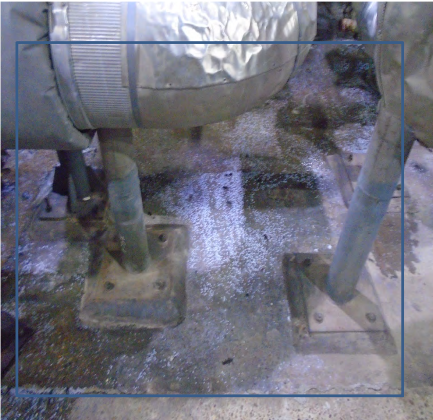
Extruder building A: Before
