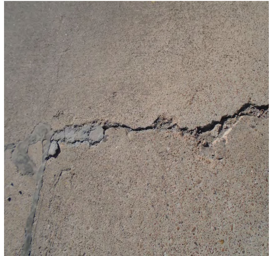
Crack between Product & Blending silos: After
